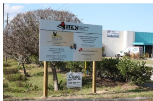
Final touches are being completed on a new office for the ELC of Marion County thanks to a great community collaboration.
